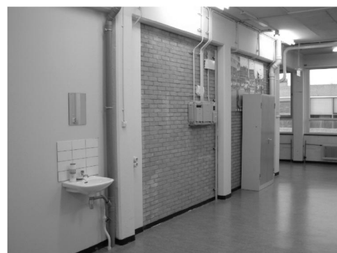
FIG. 18. Photograph of the corridor wall.
